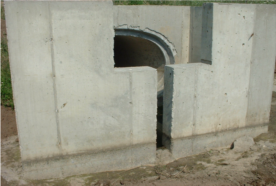
Illustration Photo #1. A concrete weir (such as the face of this catch basin) can be used to impound narrow channels.
