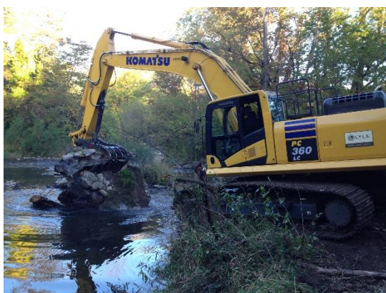
Removing Dam Remains
