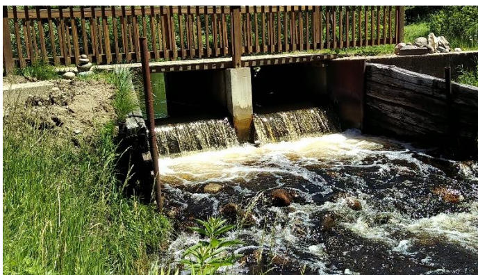
The Kinney Cr dam as seen from downstream
